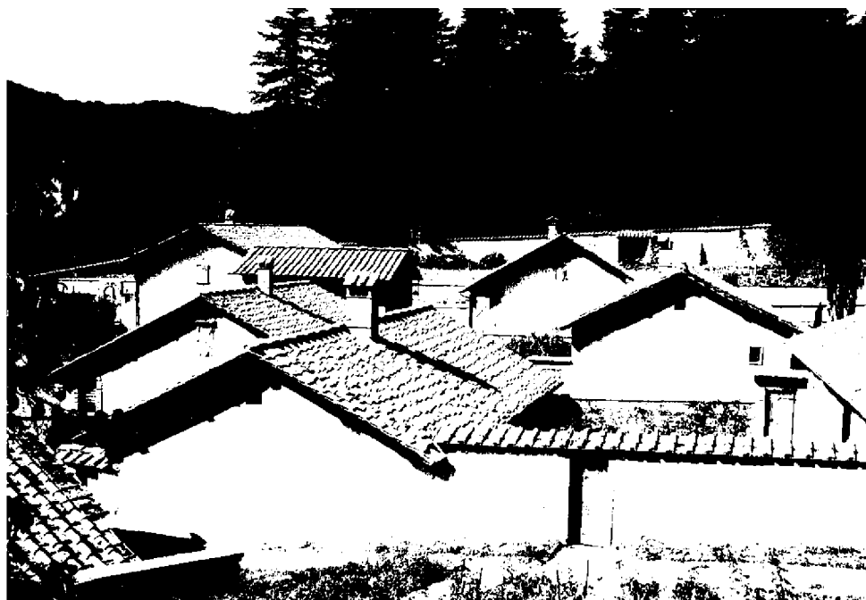
4. A view of the hermitages. In the background is the tall wall that surrounds the entire monastery grounds.
