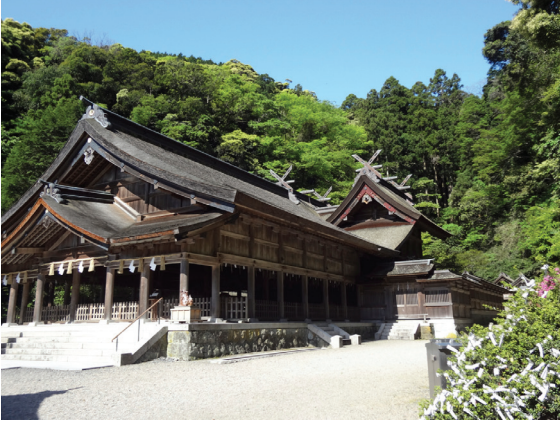
FIGURE 1. The main building of Miho Shrine.
